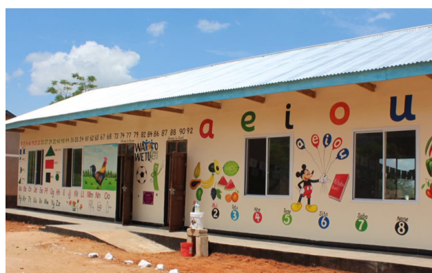
Newly constructed PPE classroom
